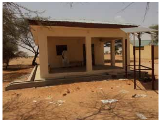
Rehabilitated facility with solar panel, Yobe
